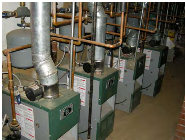
Typical dwelling unit heating boilers.
