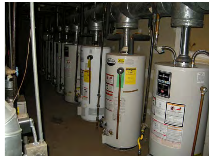
Typical dwelling unit domestic hot water heaters.
